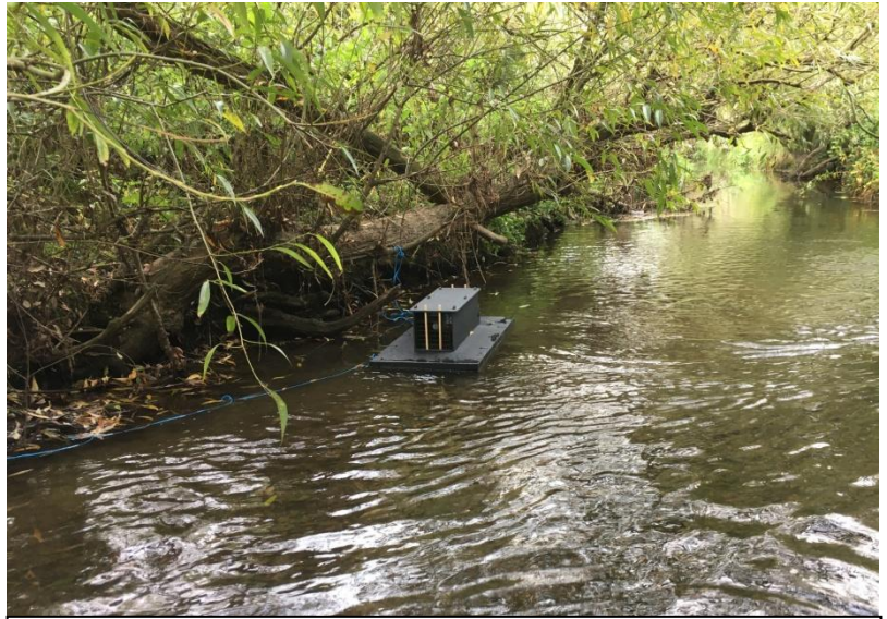
Newly installed WRT smart raft at Chelmsford in Essex
